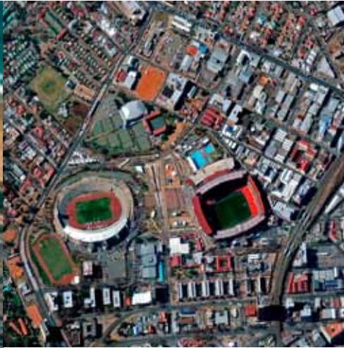
Ellis Park Stadium, Johannesburg
