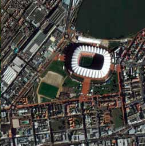
Nelson Mandela Stadium, Port Elizabeth
