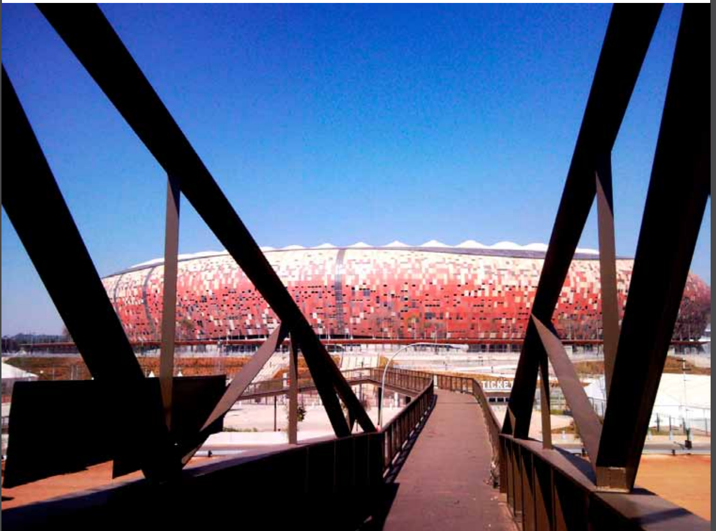
Fig 1.2. View of stadium from new bridge
