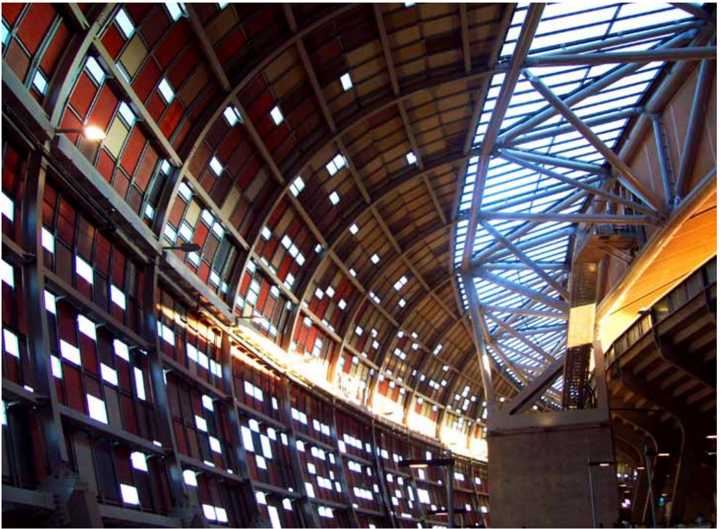
Fig 1.4. Internal view of stadium patchwork skin
